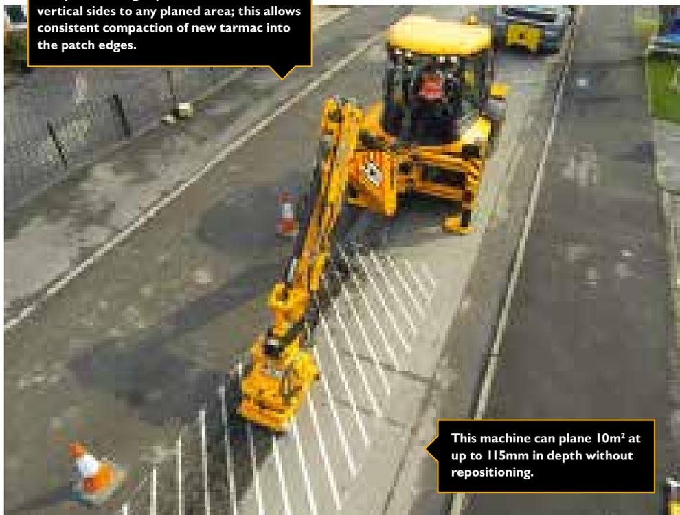
This machine can plane 10m<sup>2</sup> at up to 115mm in depth without repositioning.
